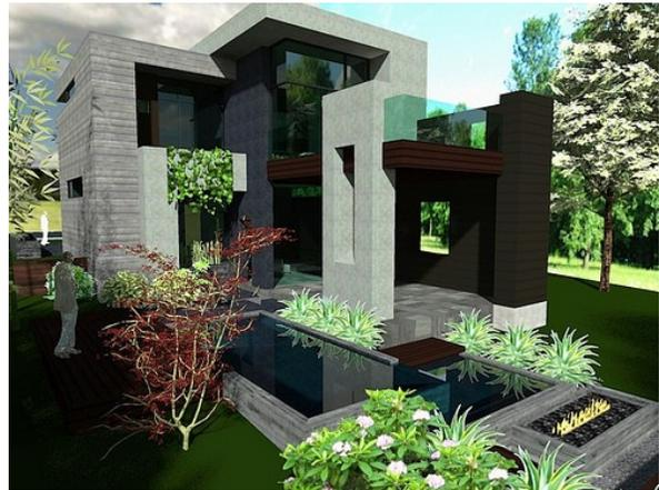
This modern residence features 6 different siding materials to include stucco, Hardi products, natural stone veneer, hardwood decks, a commercial grade fiber cement panel, and engineered bamboo. At selected locations, exterior wall materials will continue into the heated space of the house to emphasize architectural massing.
