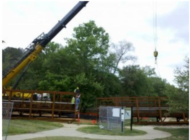
The bridge is comprised of three pieces, each weighing around 21 tons. One piece was set from the more remote side of the river, where a road had to be built in order to get the machinery to the site. The other two pieces were unloaded and bolted together on the ground on the parking lot side. Then the 42-ton double section was lifted into place. Next the third piece was lifted from the other side and the two sections were bolted in the air and then the entire bridge was set with both cranes.
