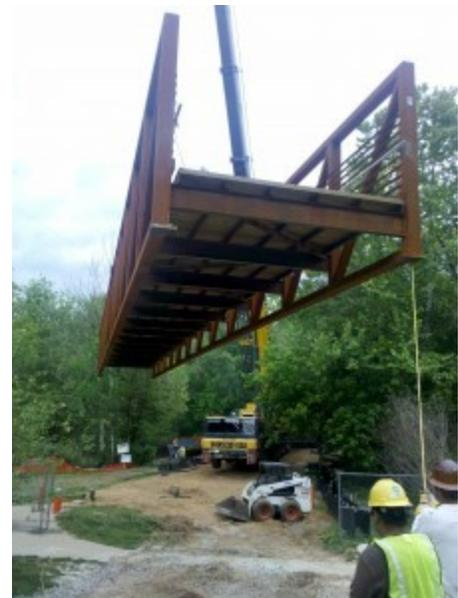
The equipment used included a 70-ton off-road crane on the remote side with dozer and excavator to make road, and a 240-ton crane on the parking lot side with 125 tons of counterweight for the big crane.
